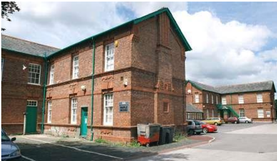
Padgate boys' houses from the south, 2001. © Peter Higginbotham.
